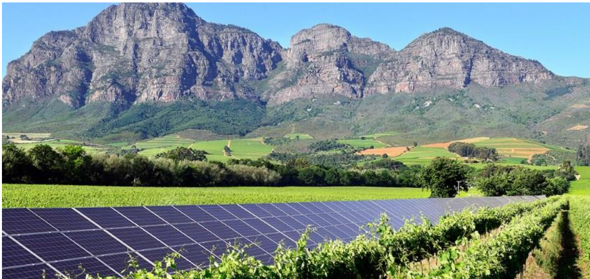
Solar PV power system on Vrede en Lust Estate
